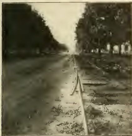
DERAILING SWITCH ON A TROLLEY LINE AT A RAILROAD CROSSING.
